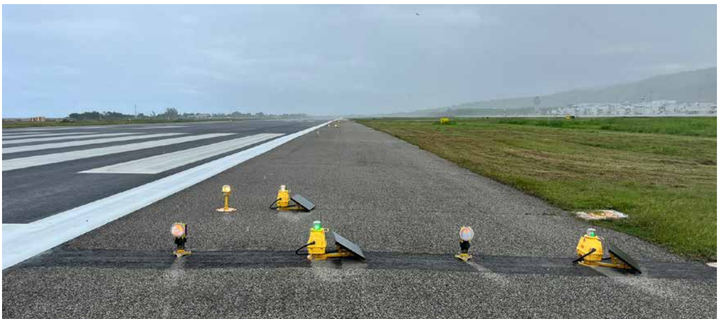
S4GA solar airfield lighting at Sangster International Airport
