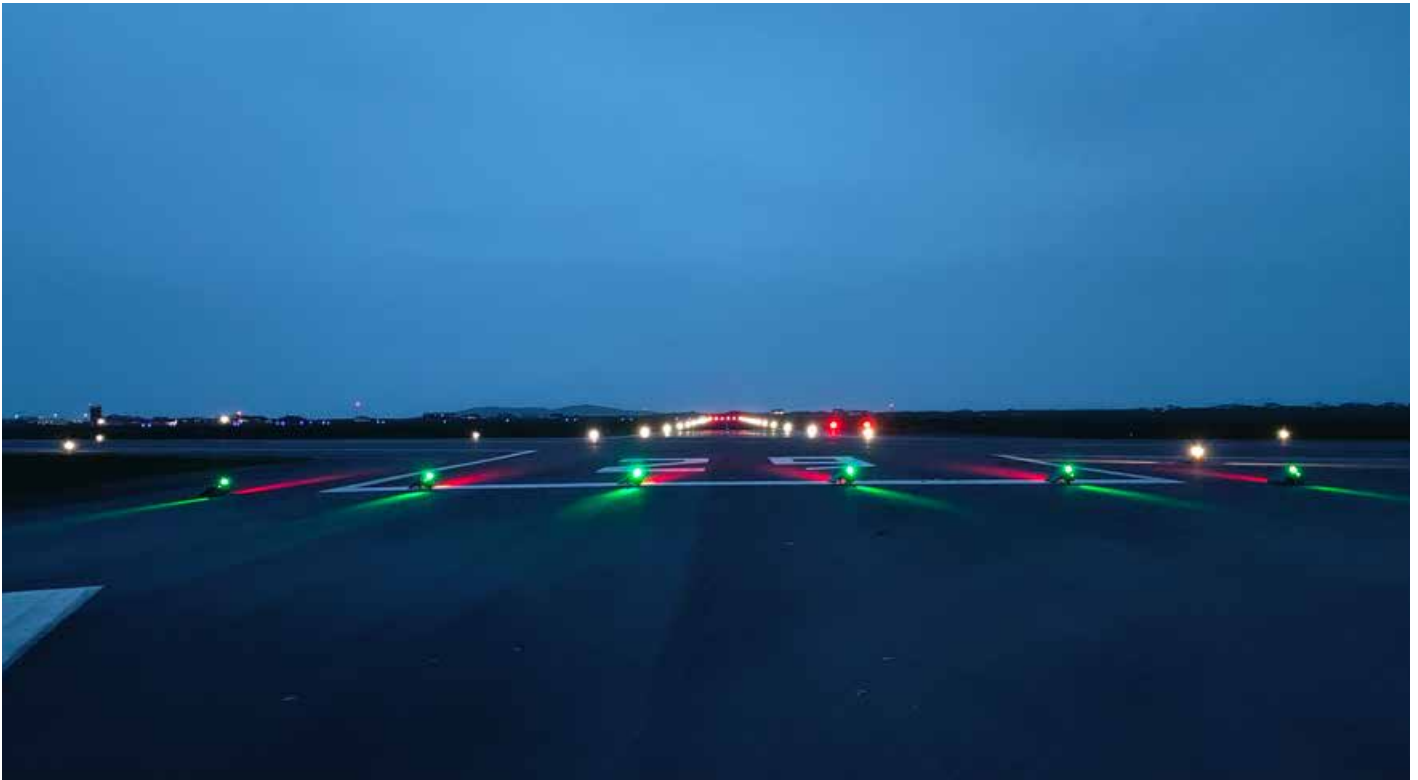
S4GA fixed solar-powered airfield lighting system
